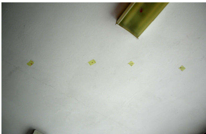
Rys. 6. Points marked on the ceiling at 15.00
