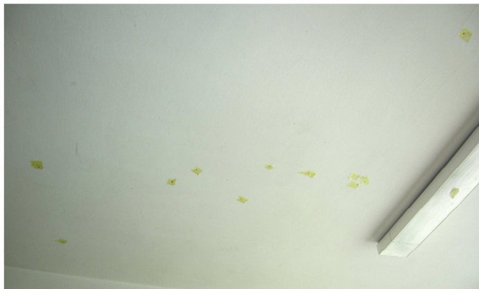
Fig. 5. Points marked on the ceiling at 12.00
