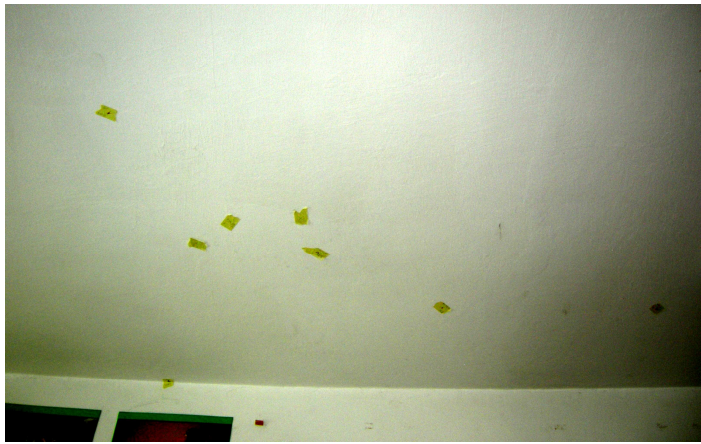
Fig. 4. Points marked on the ceiling at 8.30
